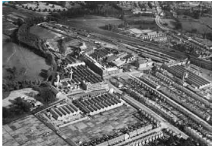
Industrialised Chelmsford Courtesy of www.britainfromabove.org.uk © English Heritage
