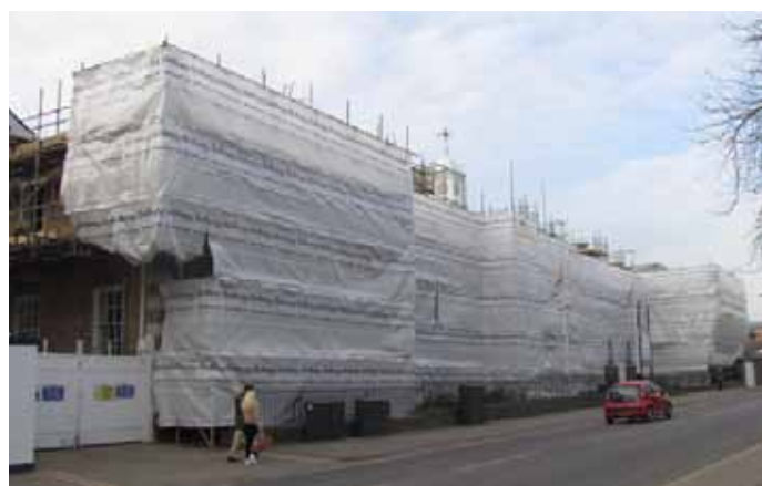
All wrapped up - the Marconi works being regenerated for housing and office space (February 2013) Rory Walsh © RGS-IBG Discovering Britain
