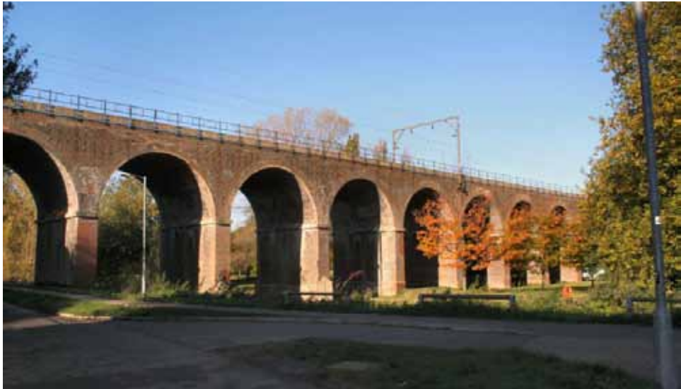
A section of the Chelmsford viaduct in Central Park © Stuart Axe via Wikimedia Commons
